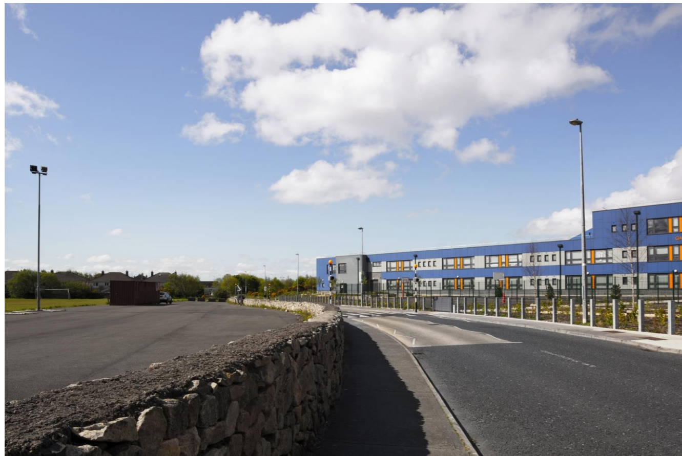
VIEW POINT 9B – EXISTING PHOTOGRAPH
